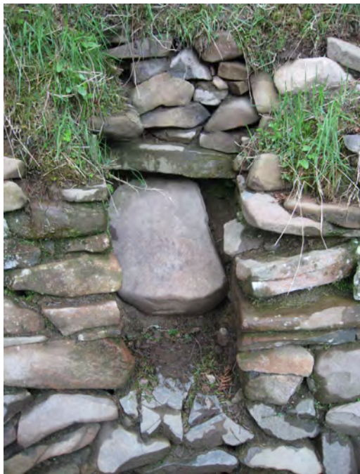
3 The fallen lintel stone at the back of the flue.
