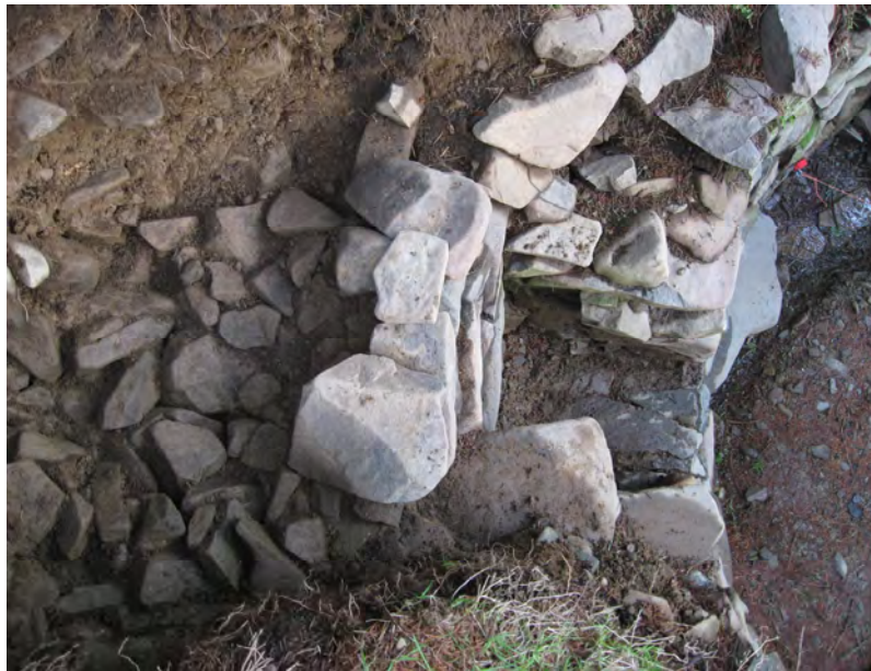
Fig7 The flue with retaining wall and stones of smoke-away viewed from above.
